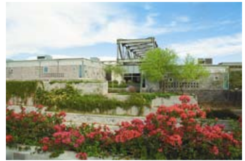
Solid Waste Transfer and Recycling Center in Phoenix, AZ
